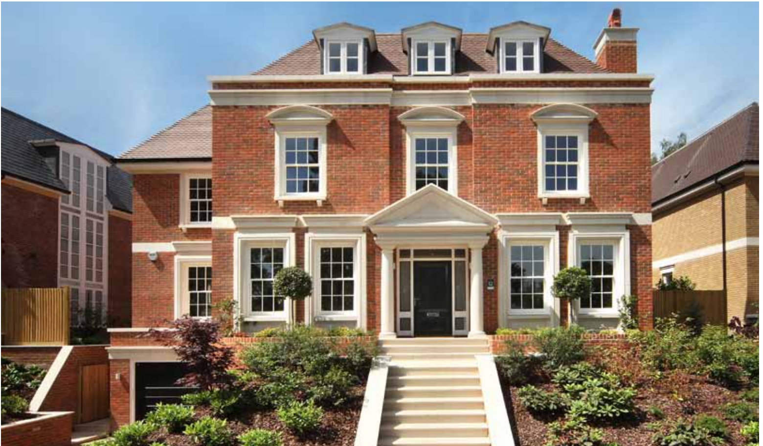
Haddonstone works closely with major architects and developers to create custom residences. Shown is part of the Wootton Place project by Octagon Developments in Esher. All the stonework is by Haddonstone.
